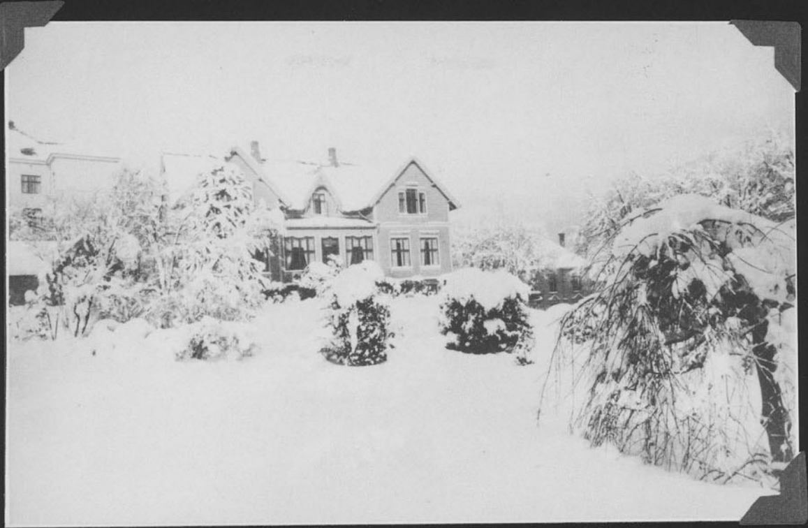
Allegaten 33. The home of V. Bjerknes and family (lower floor). The work place for the Bergen meteorologists (upper floor).
